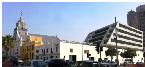
Martin Melck Warehouse Redevelopment
